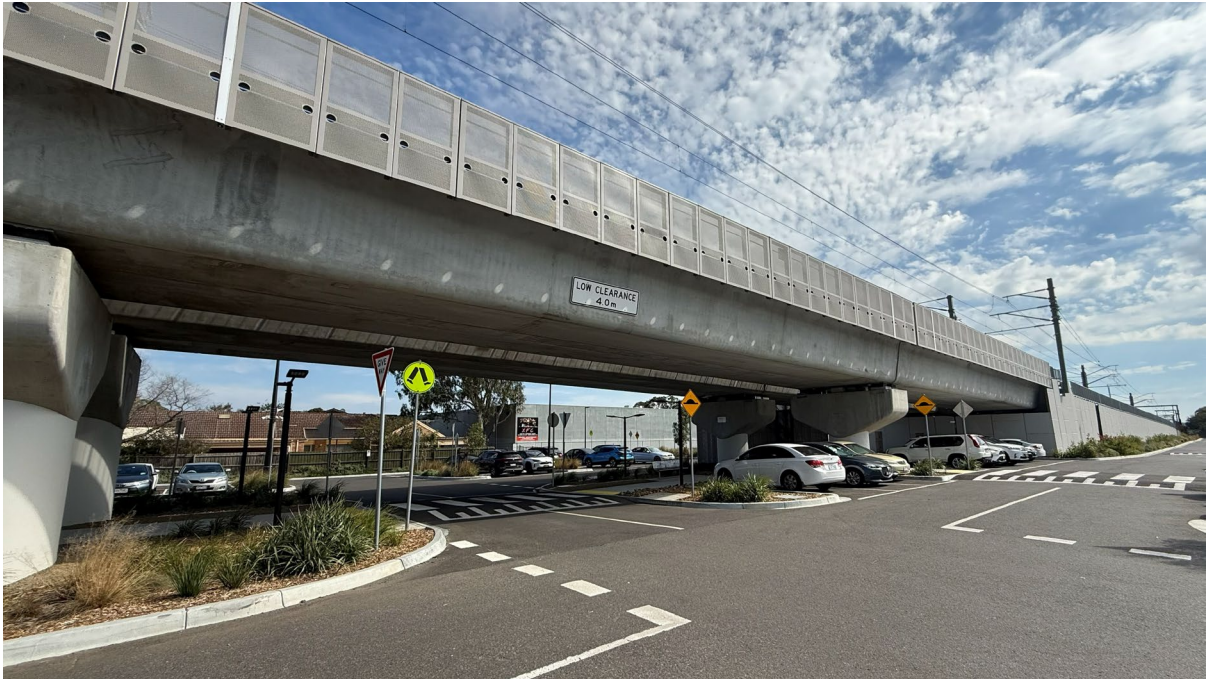
Fig. 21. Narre Warren Station precinct (Victoria) – example of a dual-track rail bridge structure and abutment.
