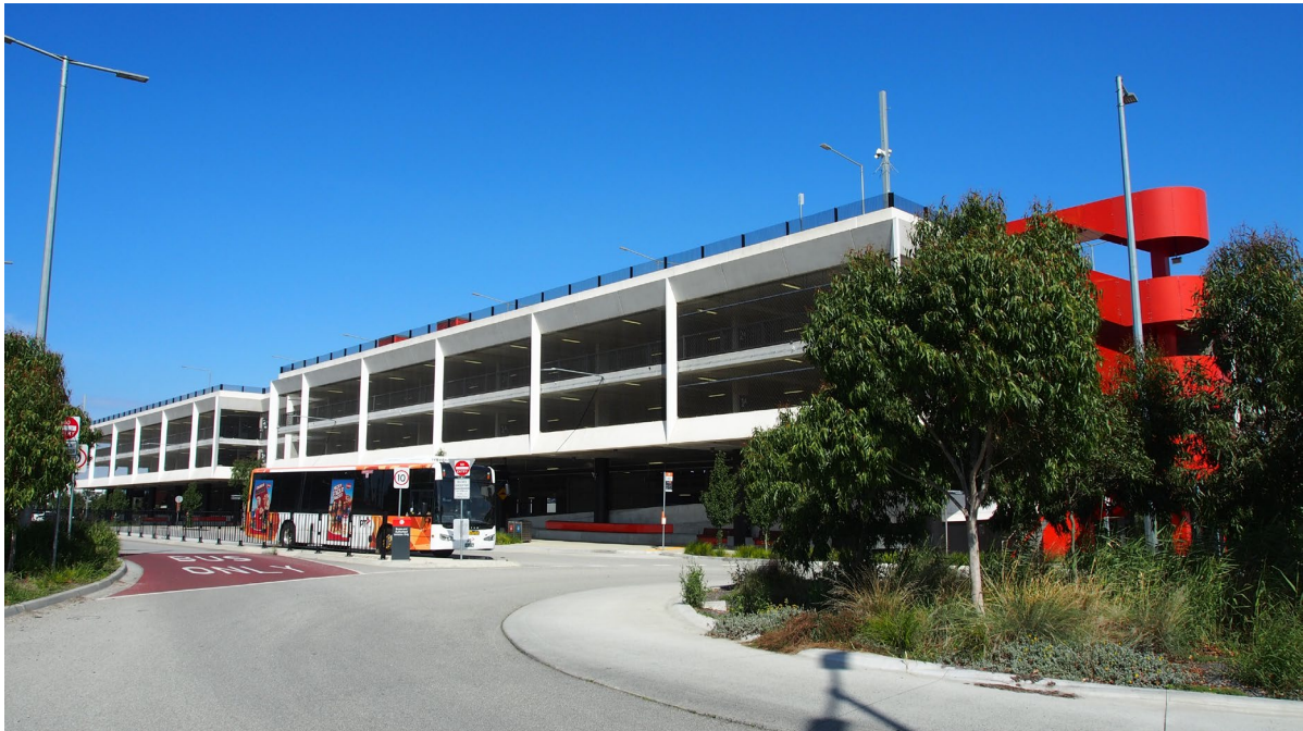
Fig. 19. Berwick Station precinct (Victoria) – example: commuter car park structure and bus interchange.
