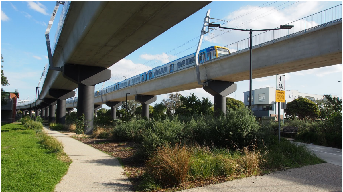
Fig. 16. Preston Station precinct (Victoria) – example: elevated railway line.
