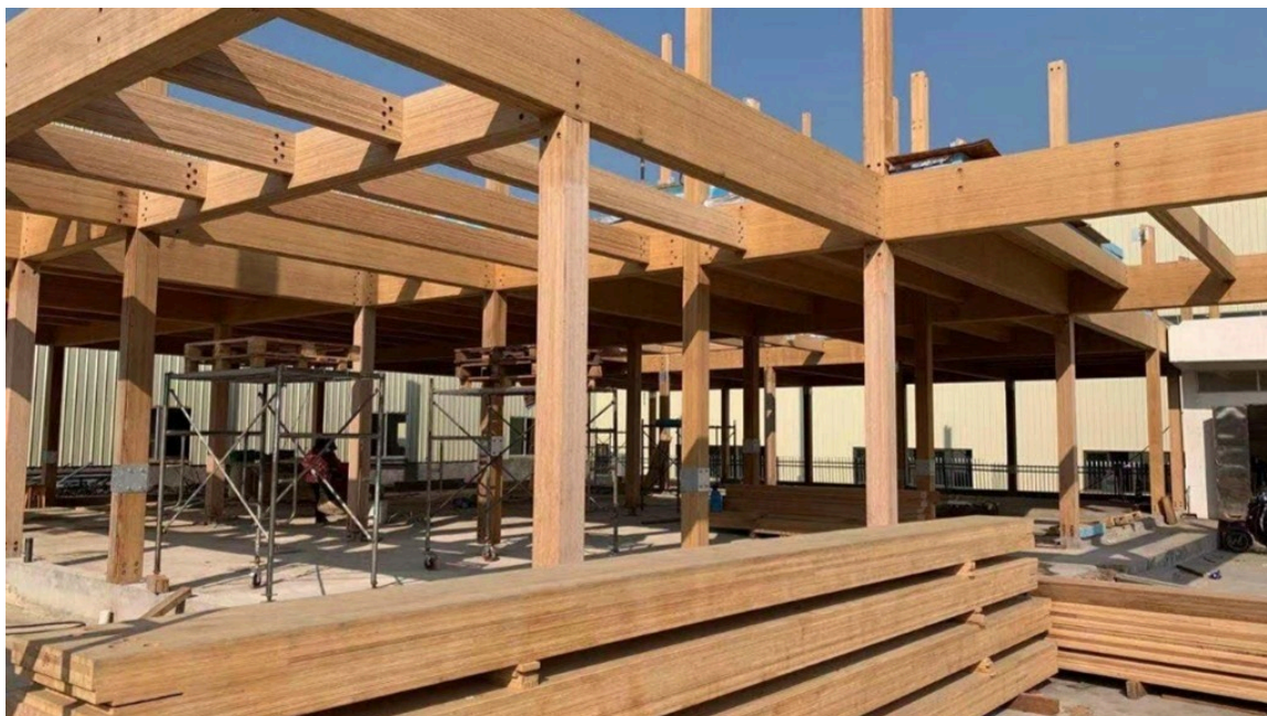
Structural bamboo construction of factory and showroom. Source: House of Bamboo
